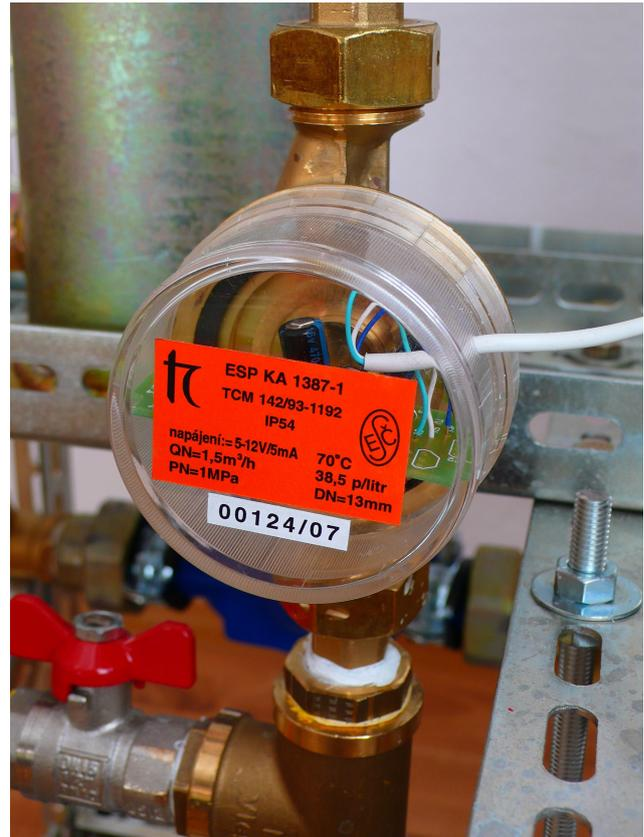
Fig. 3: Trasco – KA1387-1 flowmeter.
